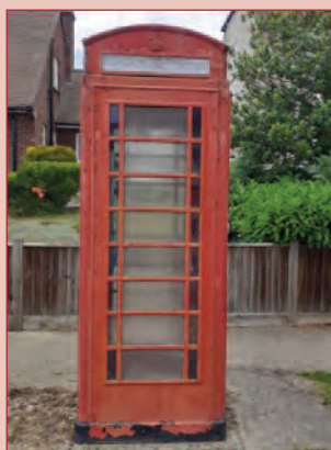
Kiosk before refurbishment:
